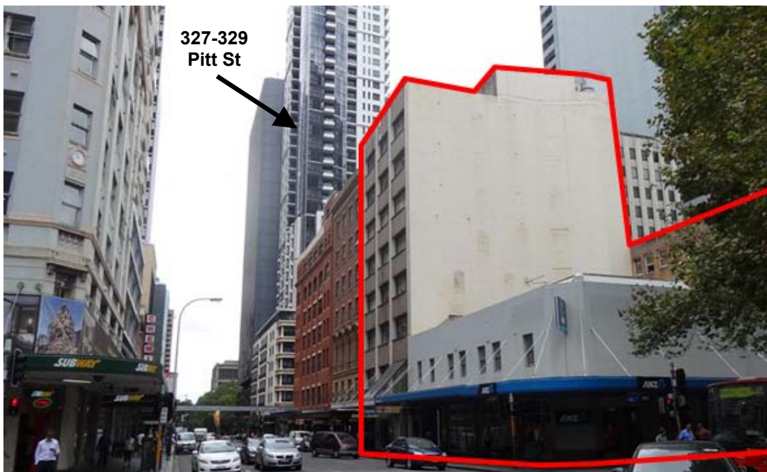
Figure 16: Castlereagh Street frontage, site (right) with 327-329 Pitt St to the west.
